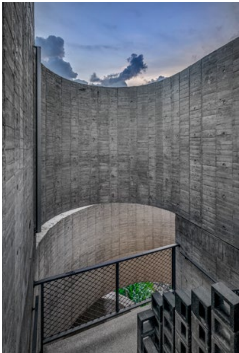
The 'flying walls' at the staircase where the walls are suspended above each other. Photography: Kuo-Min Lee
