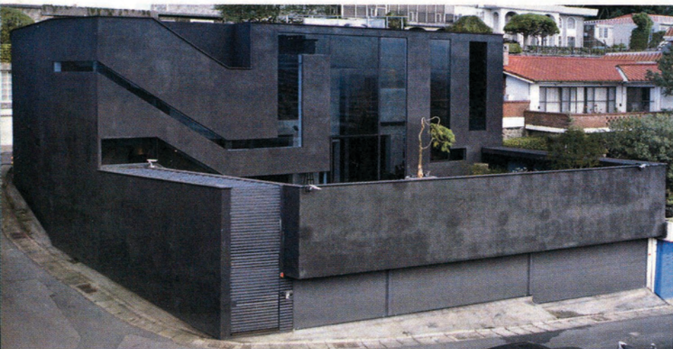
FARM LIVING: Diagonal windows add contrast to the Ant House facade. An exterior view of the house (bottom, left) demonstrates how vertical spaces lock together like "rooms" within an ant colony. The rolling deck (bottom right) opens to reveal the garage. A computer rendering (opposite) depicts how the home's additions act as a skin around the old structure
